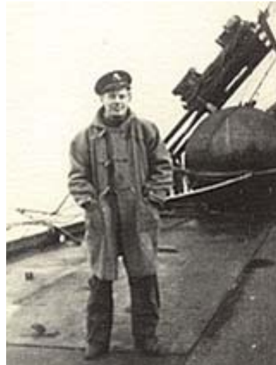
Jimmy Harland - the background shows twisted rails where tanks had rolled over the side during a gale.
