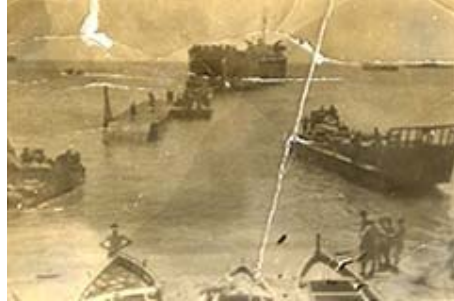
Pontoon bridge being constructed from a landing craft to the shore. From the papers of Jim Williams.
