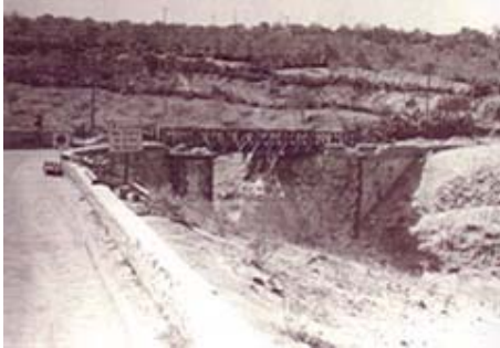
Bailey Bridge, Catania. G Wooler
